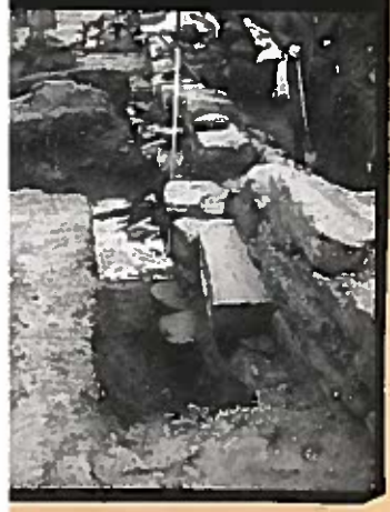
N. door (foreground) + N. wall from N.W.
