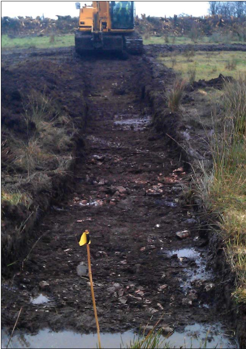
PLATE 1: Excavation in Progress
