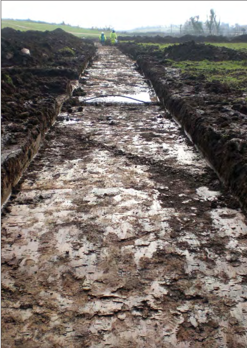
PLATE 1: TT087 under excavation
