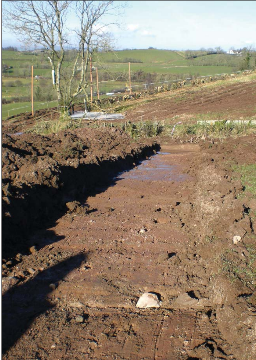
PLATE 1: TT083 under excavation
