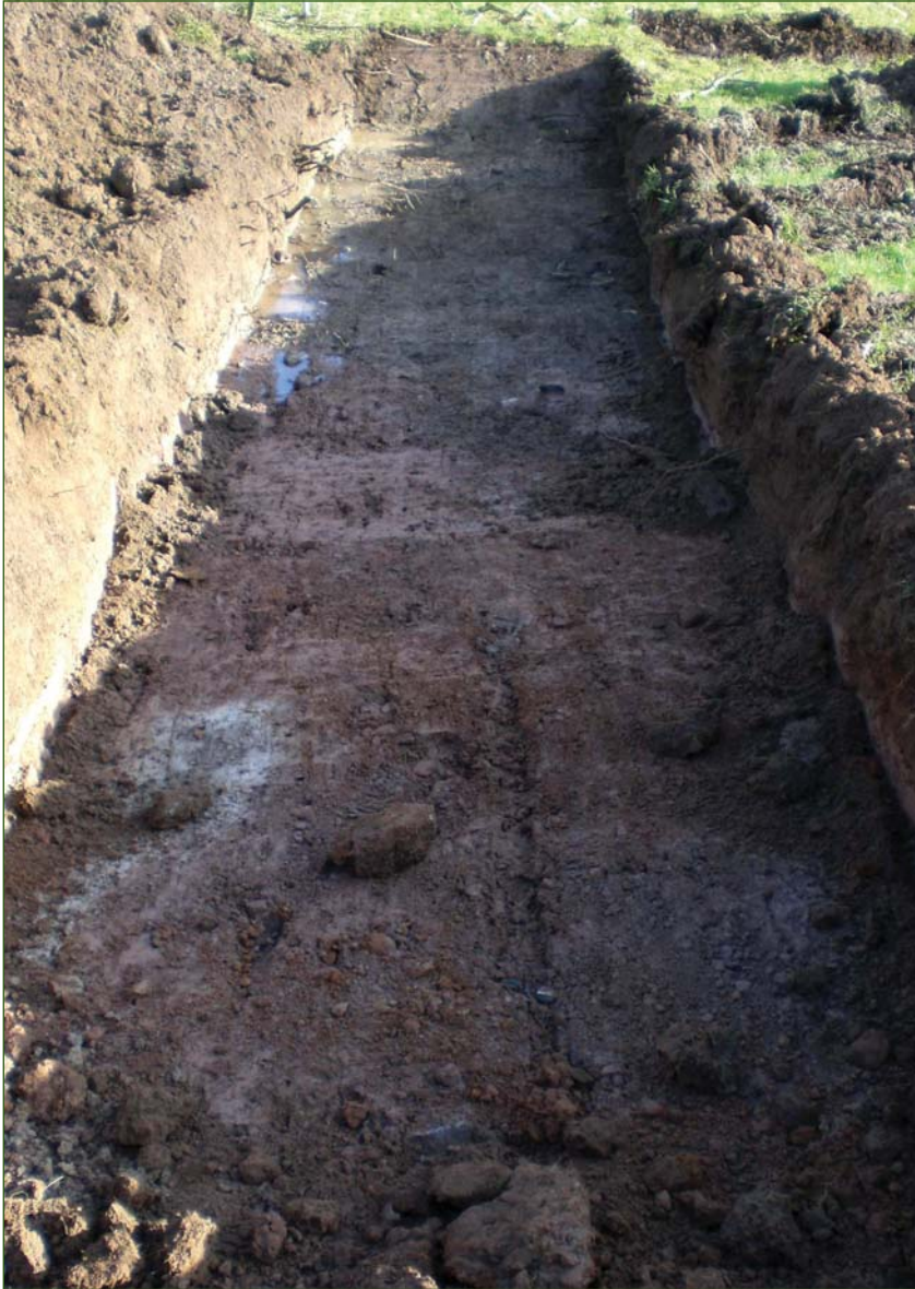
PLATE 1: TT085 under excavation
