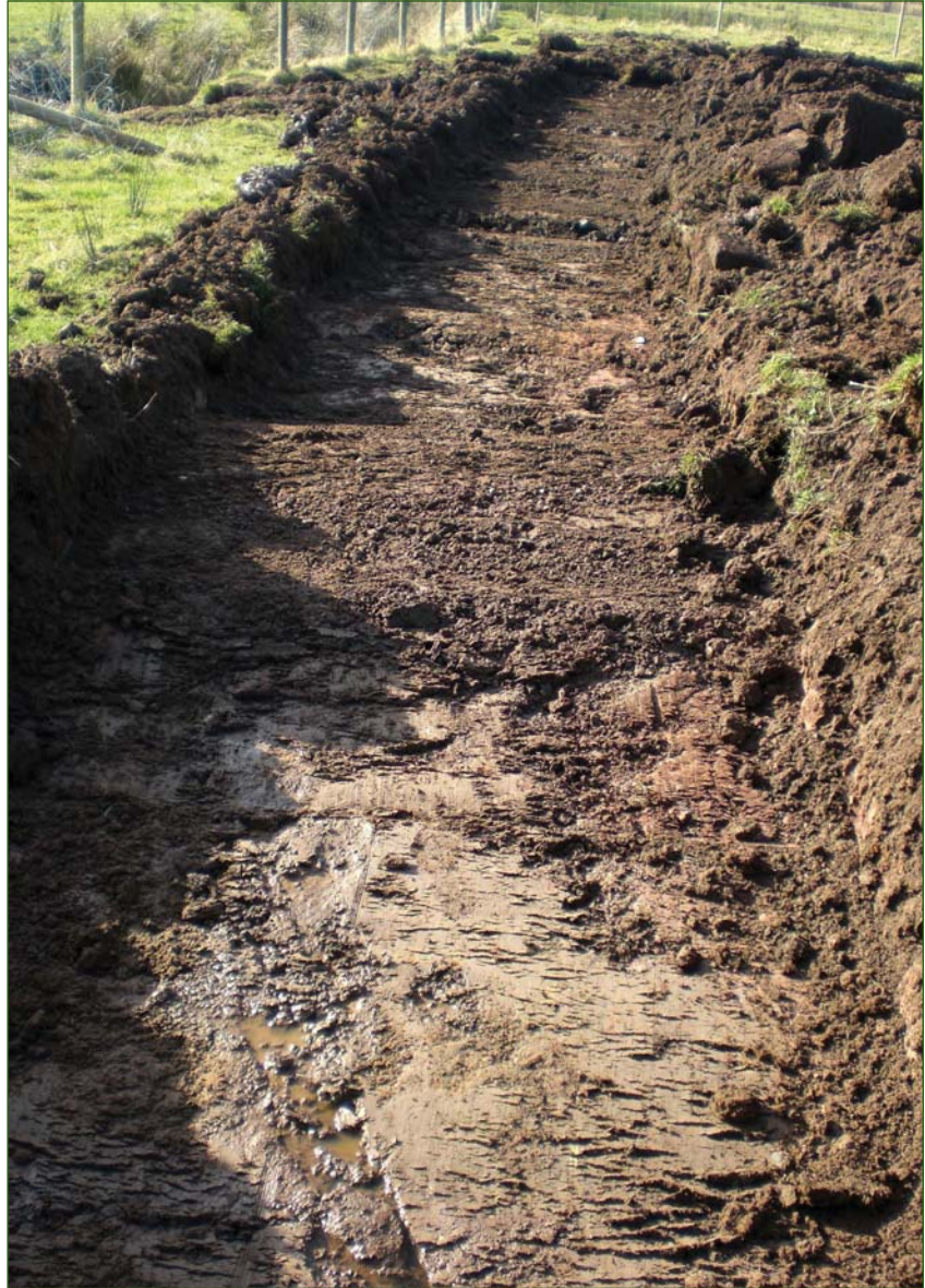
PLATE 2: TT085 under excavation
