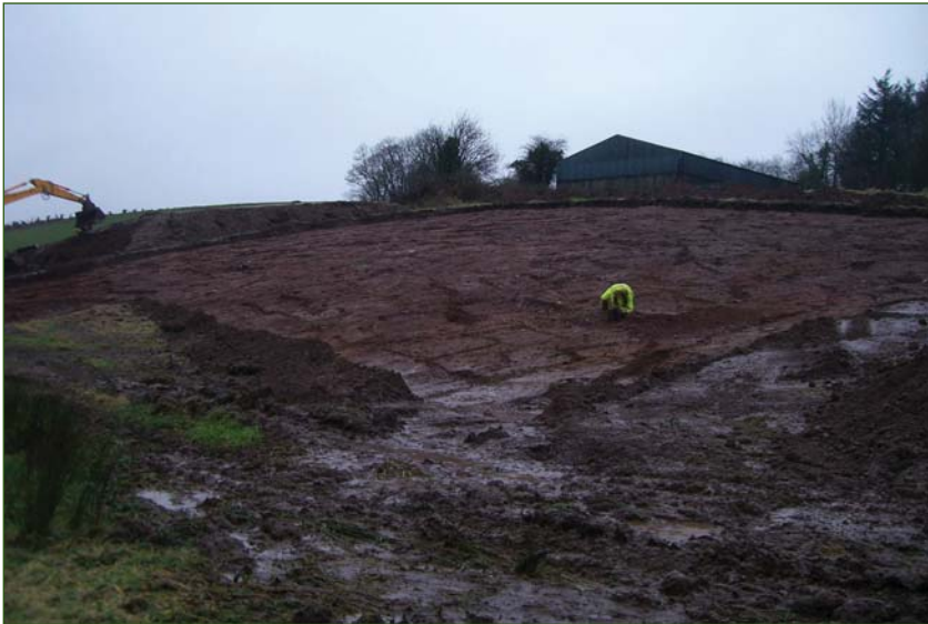
PLATE 1: SMA023 under excavation
