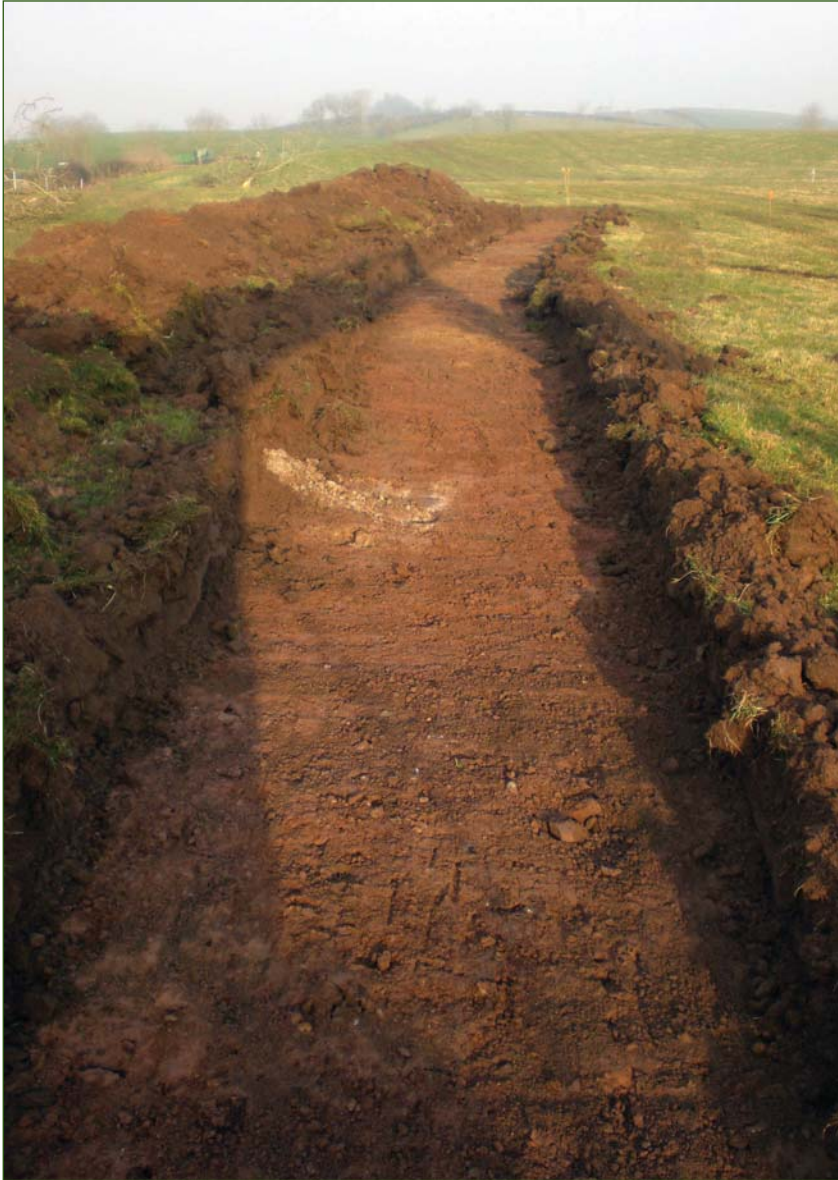
PLATE 1: TT079 under excavation
