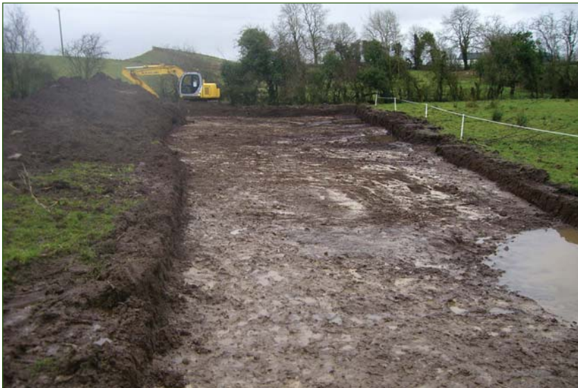
PLATE 1: SMA025 under excavation
