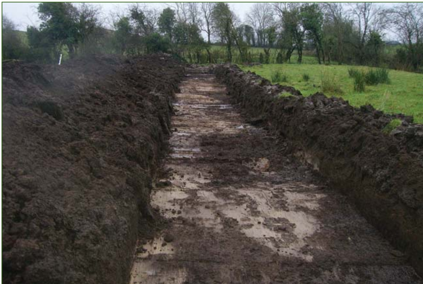
PLATE 2: Additional trench, west of SMA025; under excavation
