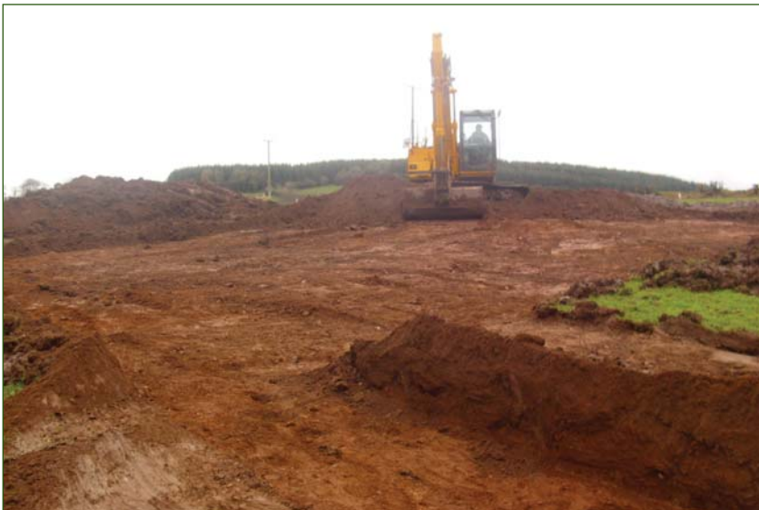
PLATE 2: SMA022 under excavation
