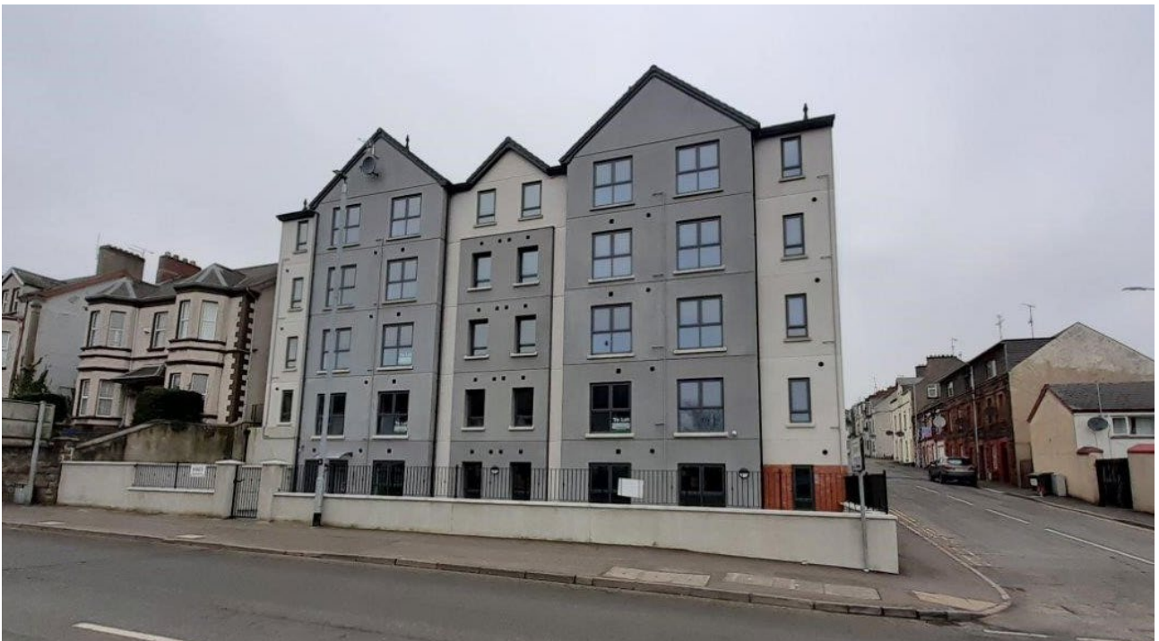
New Build Scheme – Galgorm Road, Ballymena. Triangle Housing Association, 26 Units
