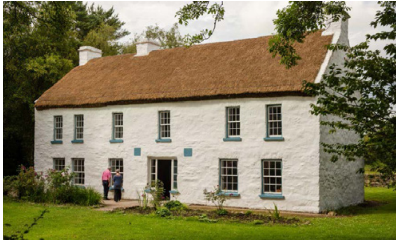
Ancestral Home of the Campbell Family, Plumbridge
