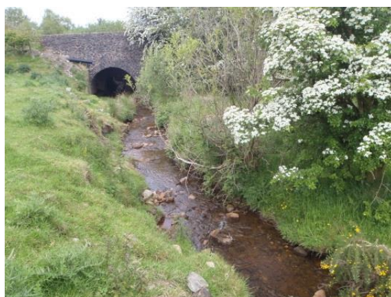
Pollanroe Burn looking downstream to Pollanroe Bridge
