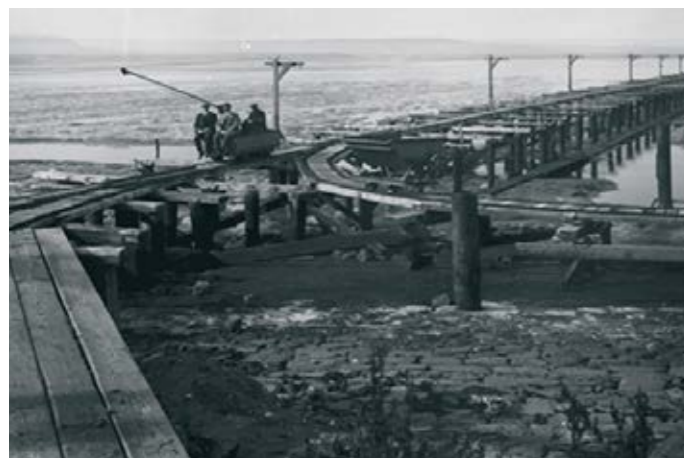
Figure 3.17 – Belfast WwTW Outfall under construction (courtesy of National Museum NI)
