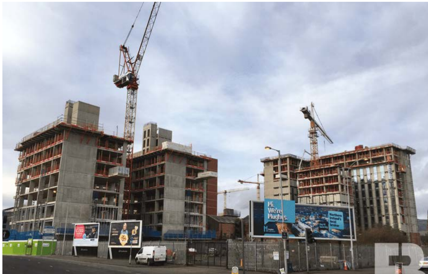
Figure 4.14 - New Ulster University Belfast Campus under construction
