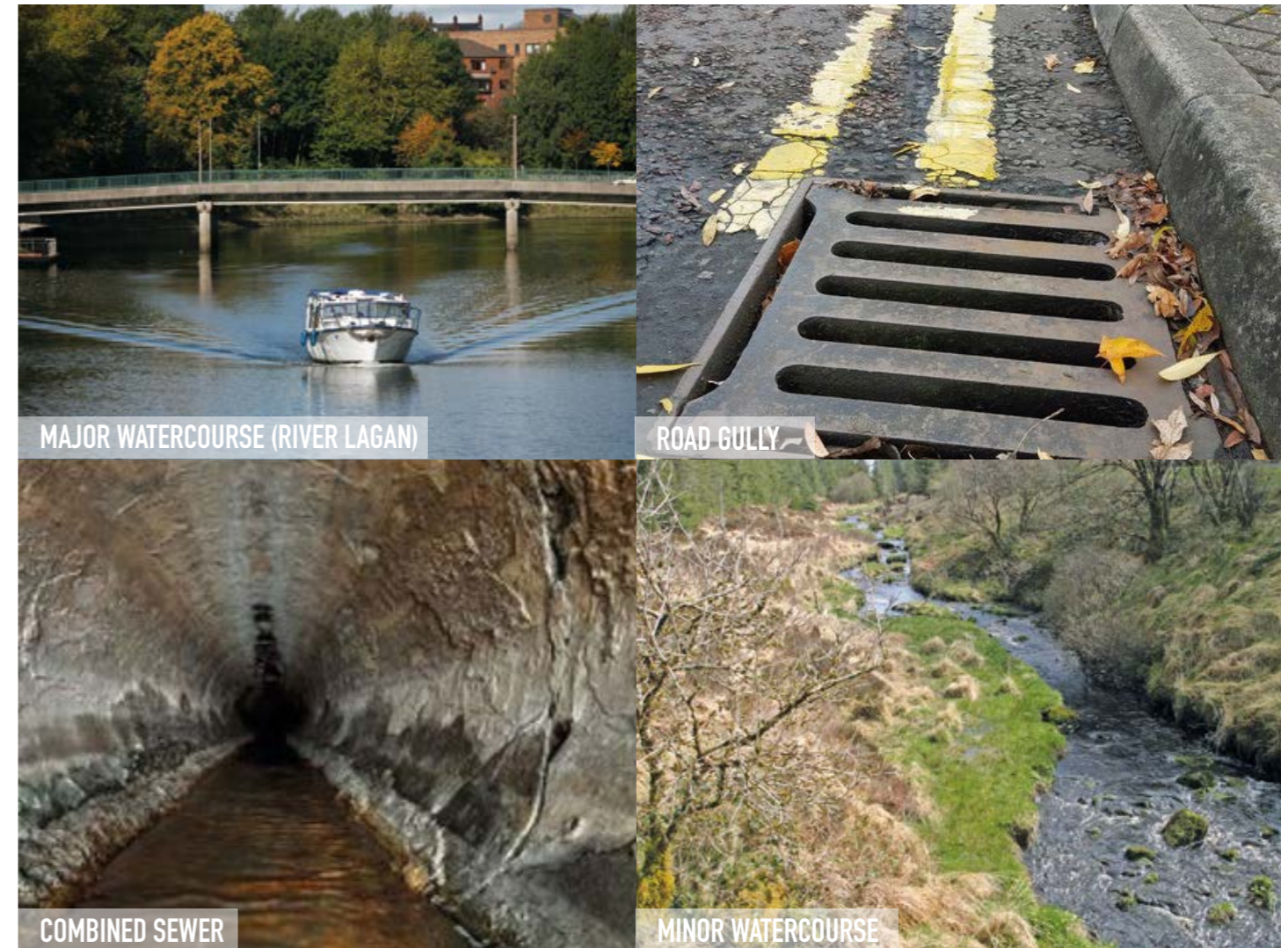
Figure 3.2: Examples of Existing Drainage Infrastructure
