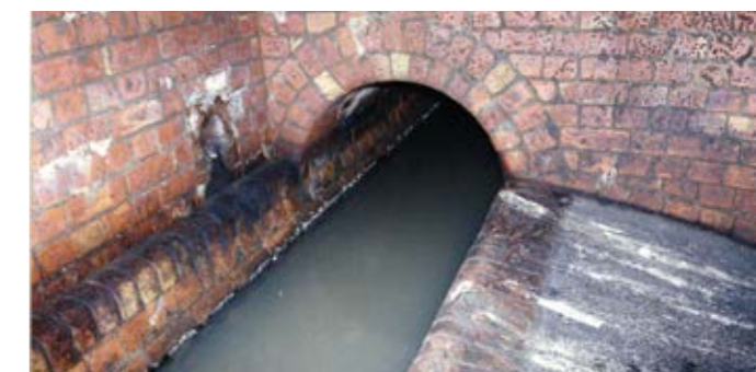
Figure 3.9 – Original Brick Combined Sewer Overflow Chamber
