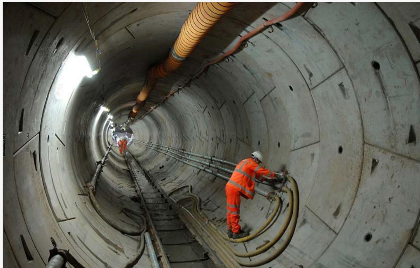
Figure 1: Belfast Storm Tunnel under Construction
