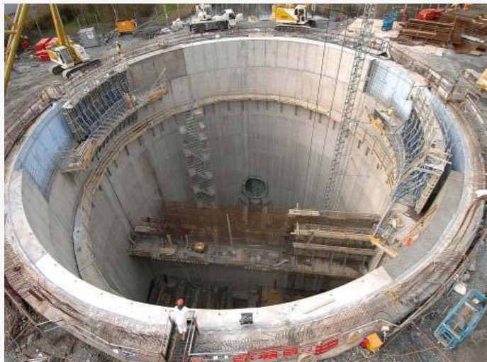
Figure 3: The Tunnel Pumping Station Shaft under construction
