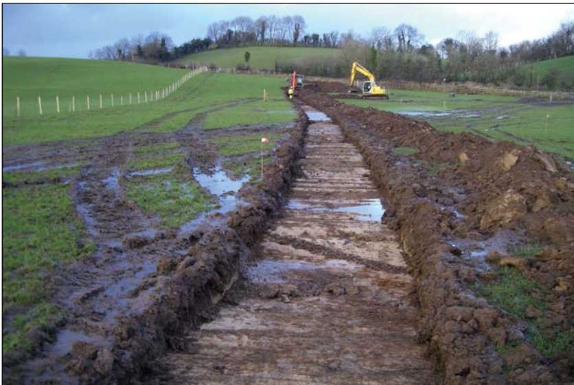
PLATE 2: TT116; Excavation in progress
