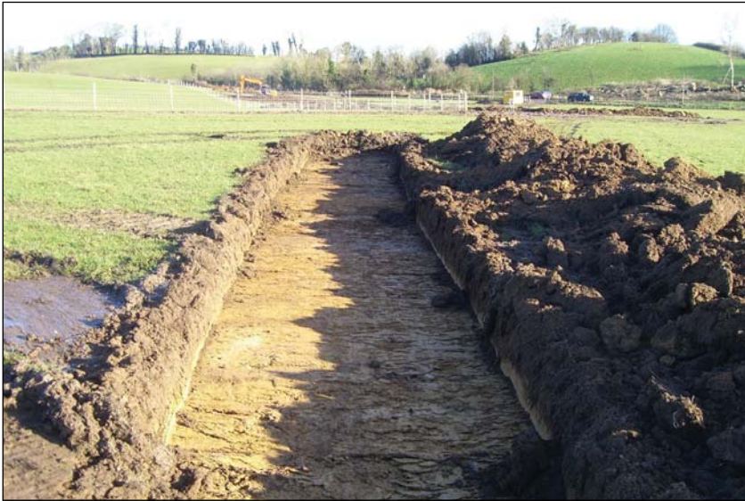
PLATE 1: TT115; Excavation in progress
