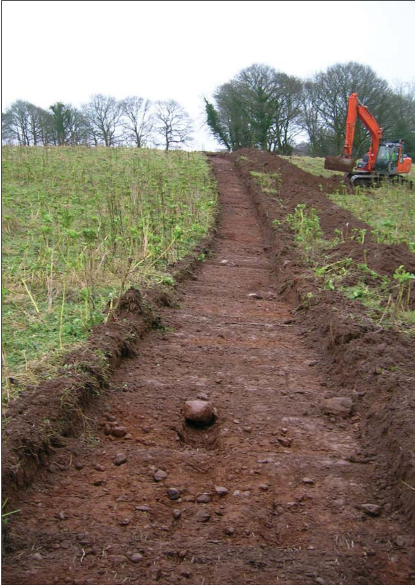
PLATE 1: TT105 mid excavation
