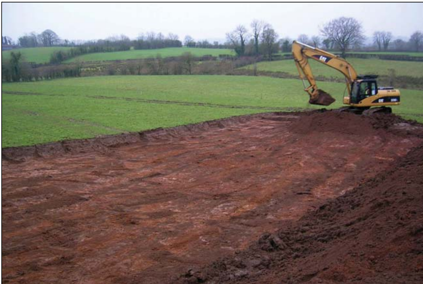
PLATE 1: SMA018 mid excavation
