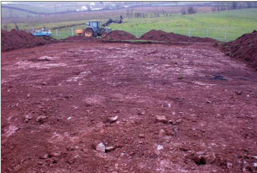
PLATE 1: SMA015; Excavation in progress
