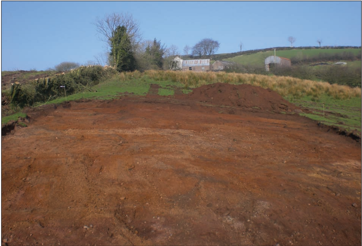
Plate 1 - SMA020 mid excavation
