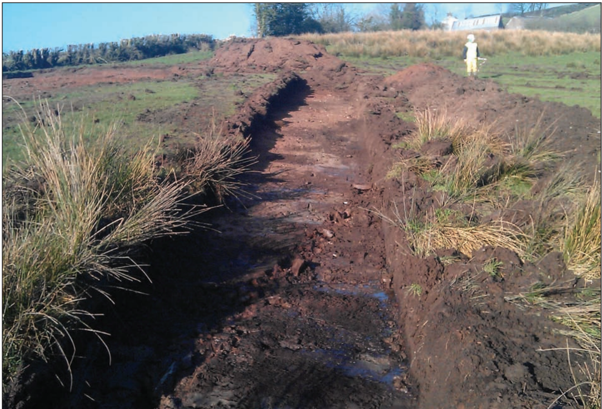
Plate 2 - SMA020 additional trenches, mid excavation
