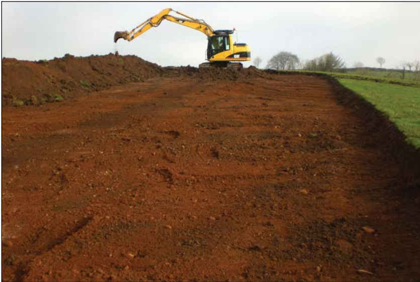
PLATE 1: SMA019 mid excavation
