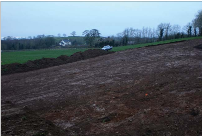
PLATE 2: SMA017; post excavation
