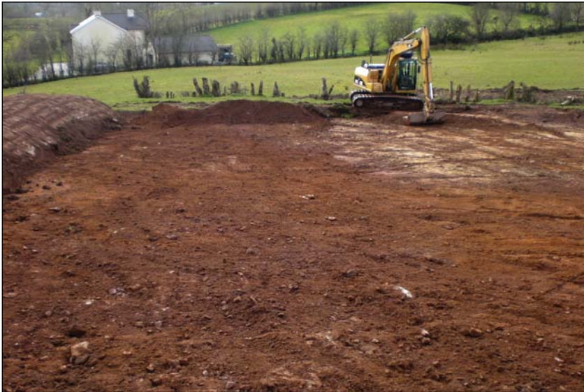
PLATE 1: SMA017; under excavation
