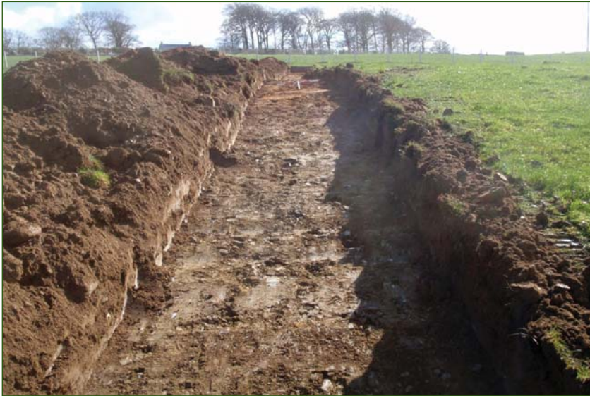
PLATE 1: TT040 under excavation
