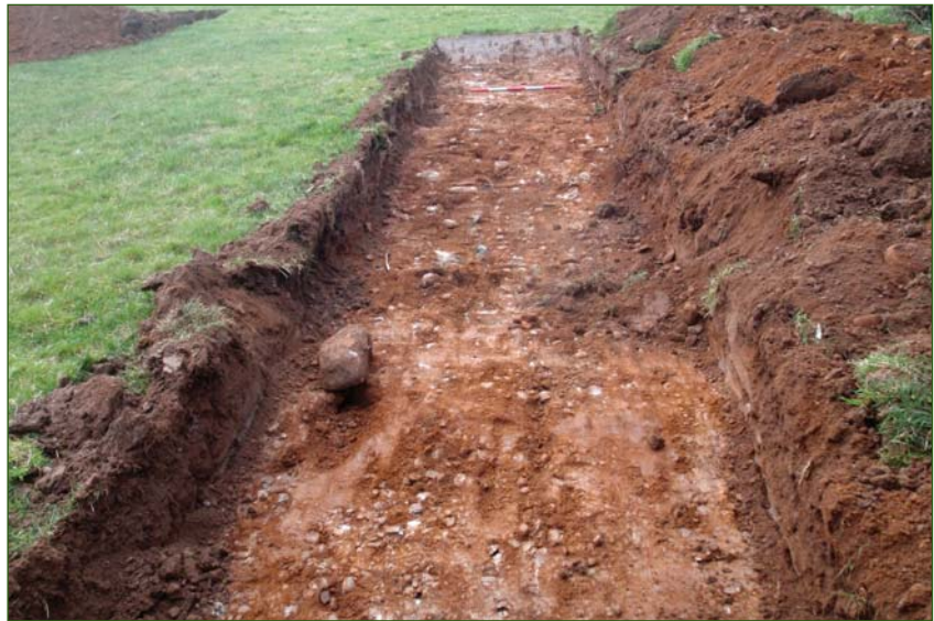
PLATE 4: TT043 under excavation
