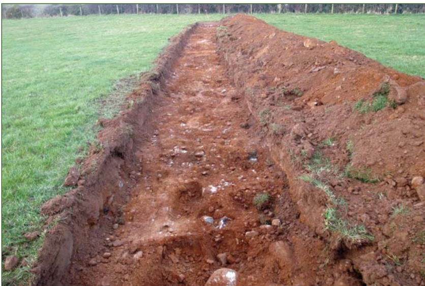
PLATE 3: TT042 under excavation
