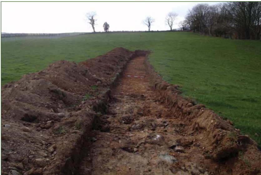
PLATE 2: TT041 under excavation
