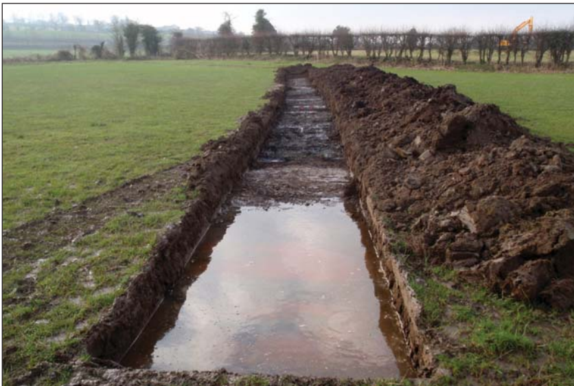
PLATE 2: TT014 under excavation
