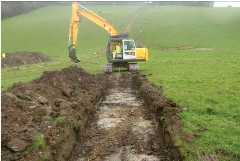
PLATE 1: TT022 under excavation
