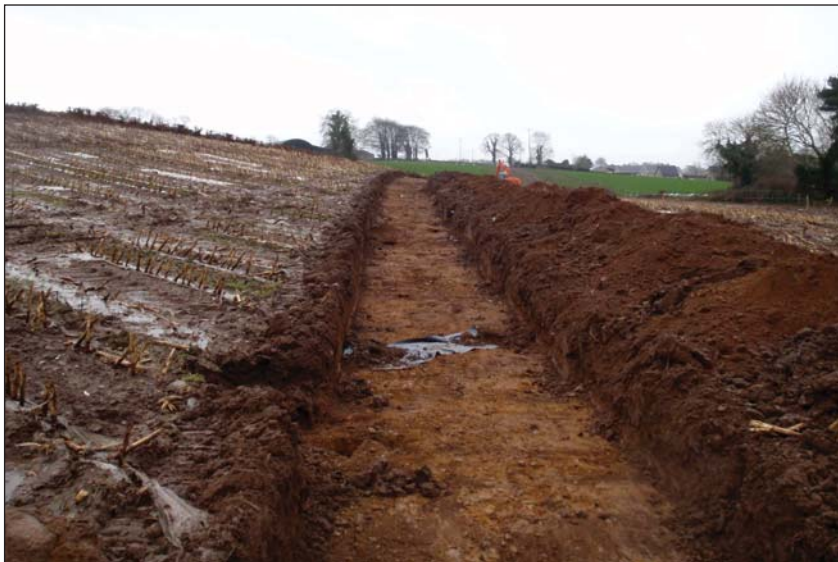
PLATE 1: TT027 mid excavation
