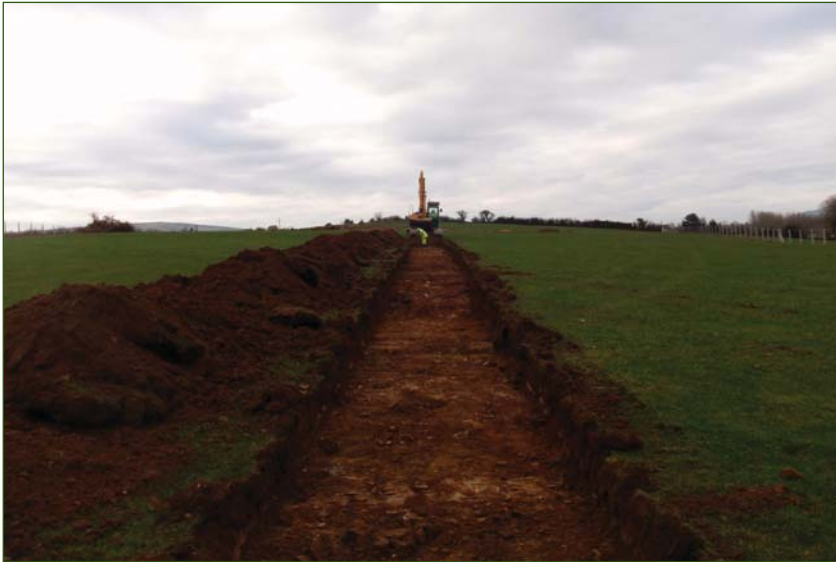
PLATE 1: TT008 under excavation
