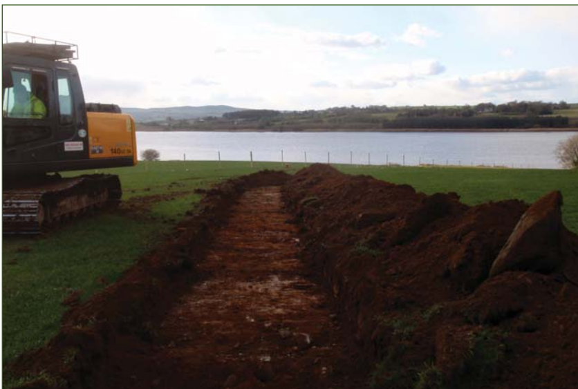
PLATE 3: TT010 under excavation
