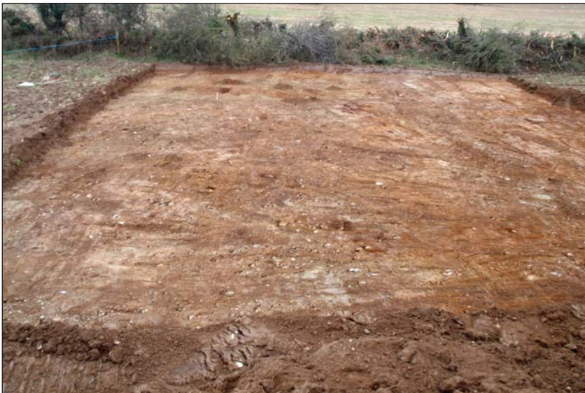
PLATE 2: SMA001 stripped; facing SW
