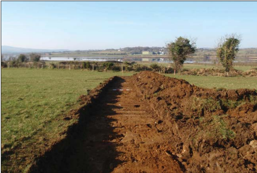
PLATE 2: AA001 under excavation
