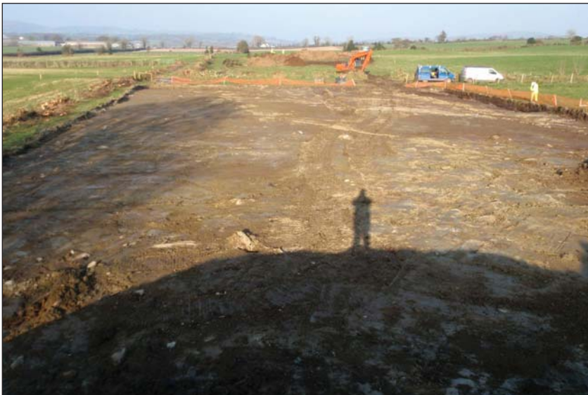
PLATE 2: SMA003 and extension under excavation
