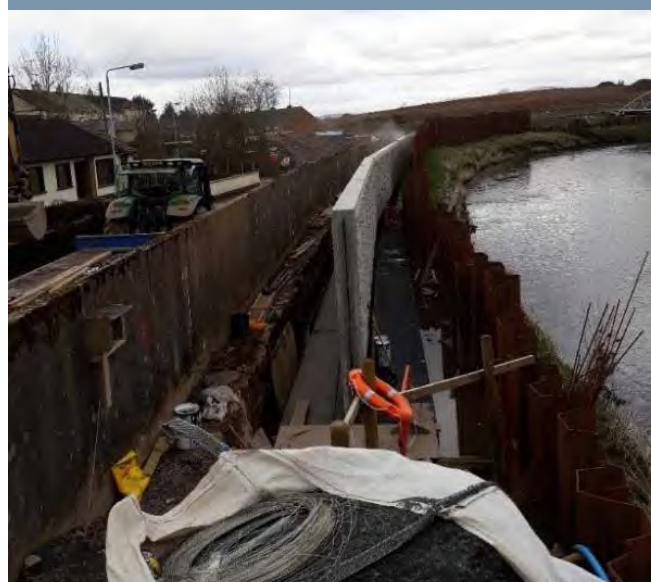
Figure 5.9-13: Floodwall construction as part of the Hunter Crescent Flood Defence scheme
