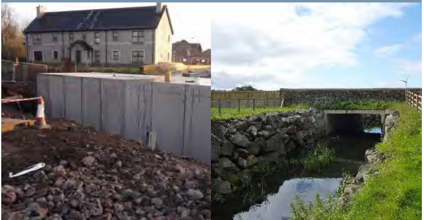
Figure 5.5-10: Photographs taken during Park Road culvert construction and of completed works
