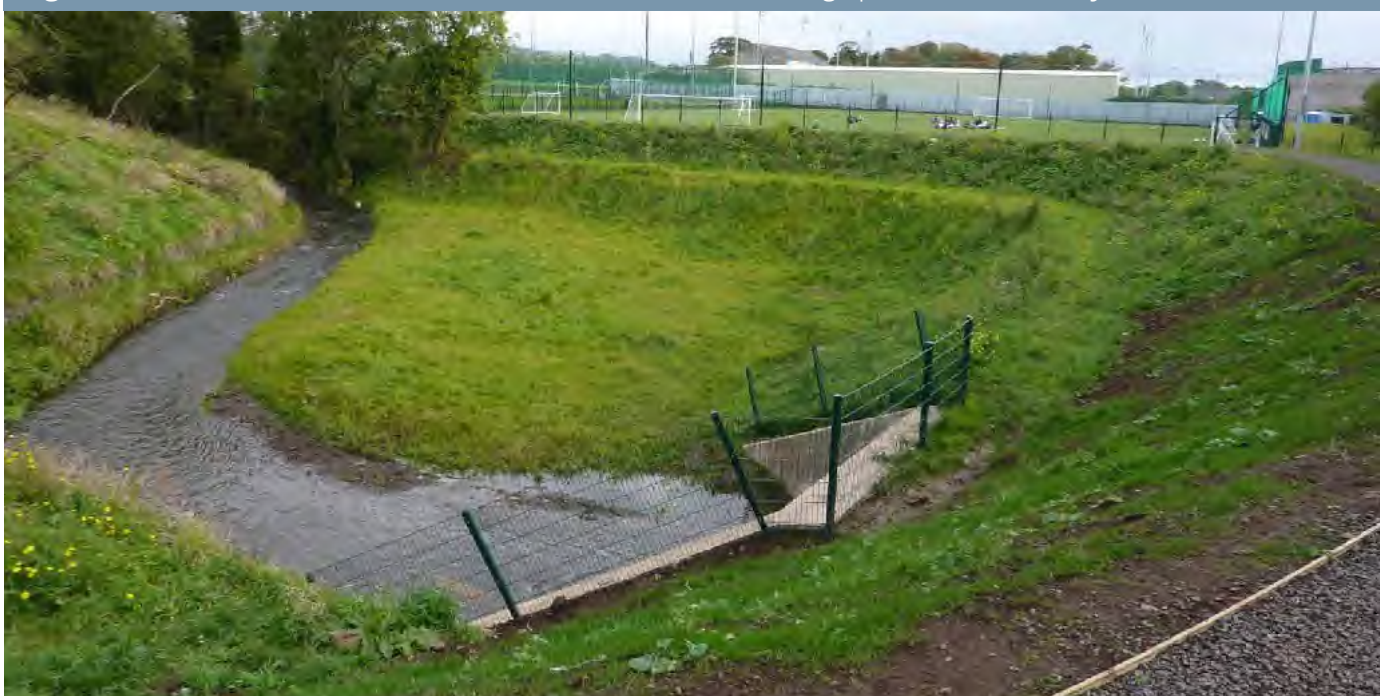
Figure 5.11-9: Sullatober Water Flood Alleviation Scheme storage pond in Shaftesbury Park
